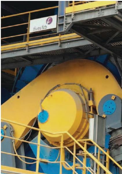
The high moisture content of the pozzolana used in Republic Cement's Norzagaray plant required a drying process, carried out by an FCB Aerodecator with hot gas from the clinker cooler exhaust used to reduce the moisture content of the pozzolana
