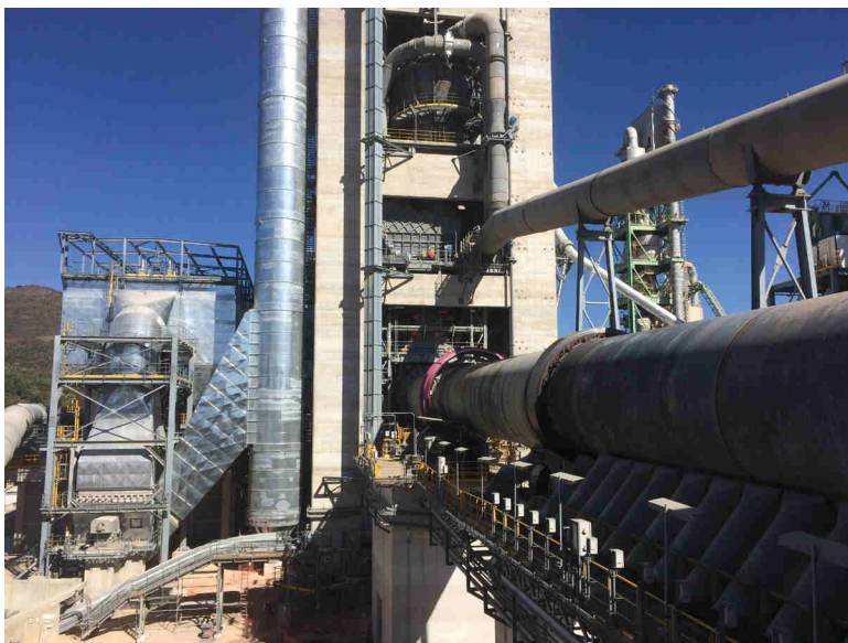
Figure 10. FCB Preheater and calciner with AF feeding.
