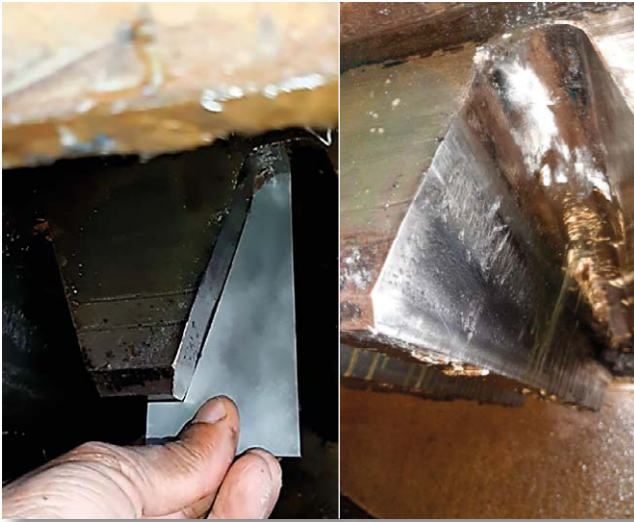
Figure 6: Low profile wear (0.4 mm), but important spalling
