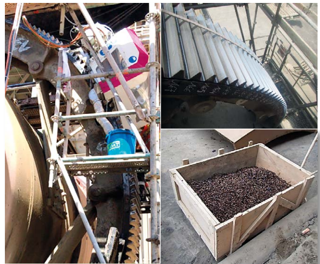
Figure 5: Machining on a rotary kiln in a cement plant in Morocco
