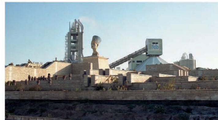
Minya - Helwan Portland Cement Co (Egypt) 750 tpd with Precalciner & Spray cooler
