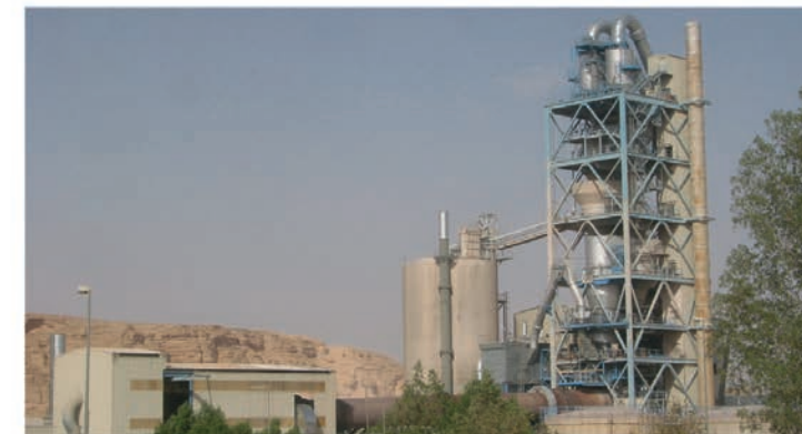
Muzahmiah - Saudi White Cement Co. (Saudi Arabia) 1,000 tpd with Precalciner & Dual cooler
