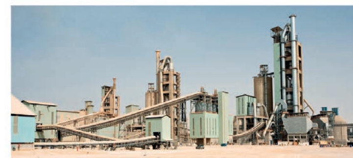
Umm Bab - Qatar National Cement Co. (Qatar) 2,000/4,000/2 x 5,000 tpd with Alkali by-pass - Natural gas
