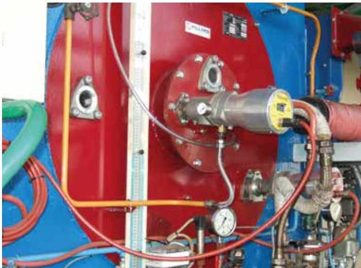
Pillard Packlight™ installed on a burner
