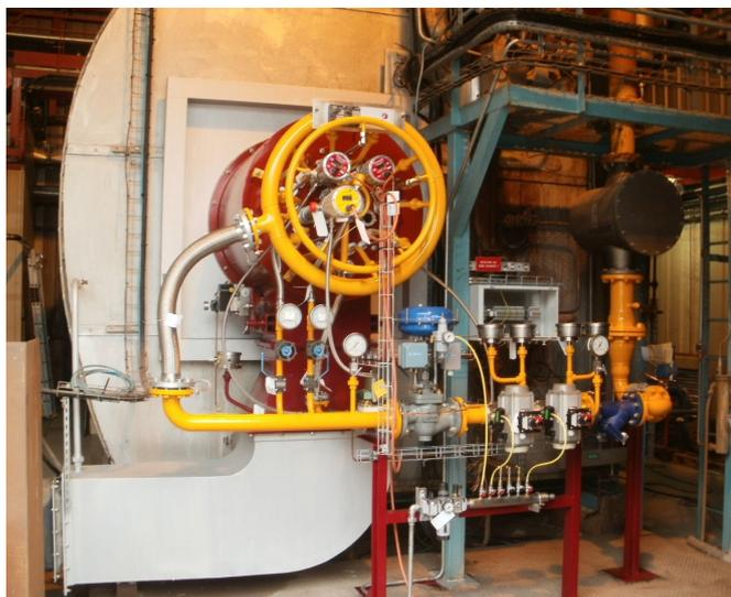
The Pillard LONoxFLAM® G2 burner has very low NOx properties for fuel gas.
