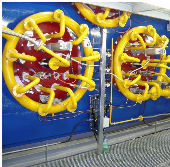
The Pillard LONoxFLAM® G2 has very low NOx properties with less than 30 ppm at 3.0% O<sub>2</sub> dry, enabling between 50 and 75% NOx emissions reduction in heating plants, sugar plants, utility boilers and refineries.
