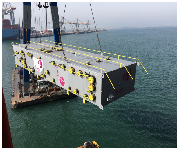
Figure 2. Cold box during its transportation to a gas treatment unit.
