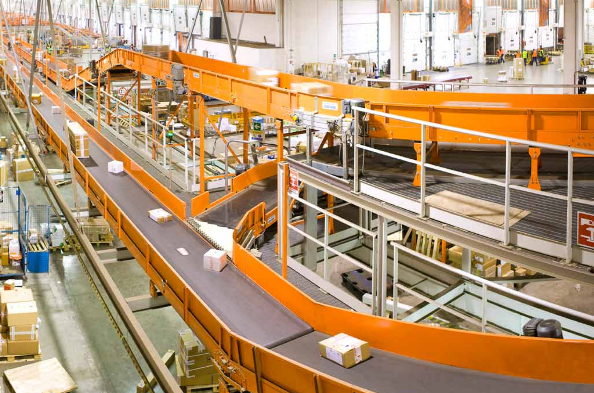
2009 | Automated parcel sorting center (Italy)
