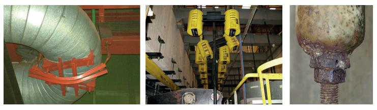
A deviation on a support may cause damages and uncontrolled events on pipes. There has to be sufficient control of supports to ensure the continuous operation of the installation.
