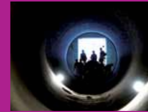
Page 16 • View of the interior of a cement plant's furnace
