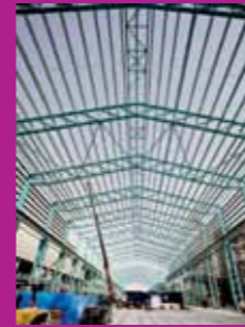
Page 14 • Aluminium plant under construction
