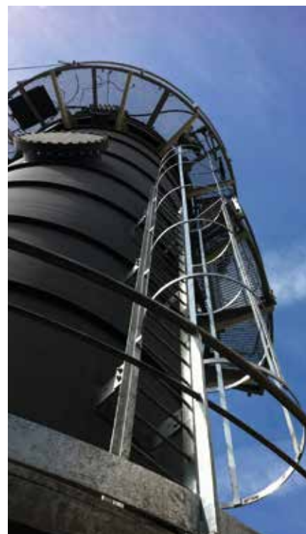
Lesaffre-Frères sugar plant at Nangis. Production: 900 tpd
